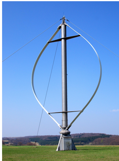
Figura 1.3: Torre eólica com aerogerador de eixo vertical do tipo Darrieus. FONTE: https://en.wind-turbine-models.com/turbines/93-dornier-darrieus-55?picture=LPQ8tvaHYVd
